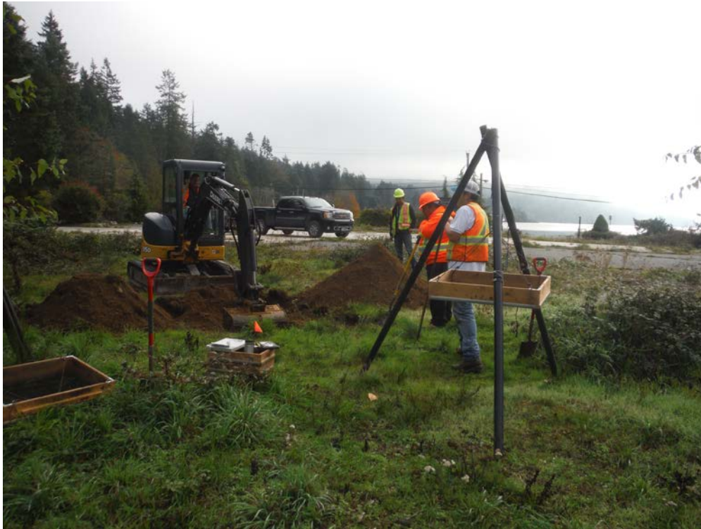
Figure 1: Project area view east at excavation and screening activities
